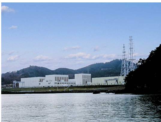
The Onagawa Nuclear Power Plant
