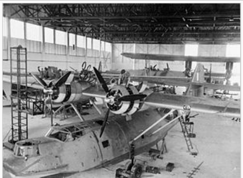
Catalina Is of 205 Sqn. RAF undergoing service in their hangar at Seletar, Singapore.
